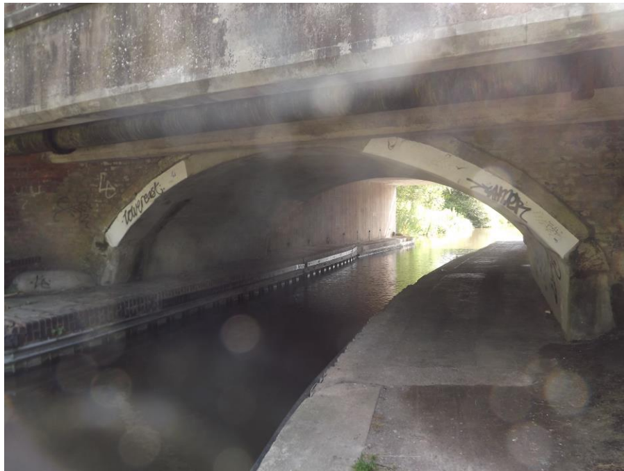
Figure 38 Radford Bridge, No.98
