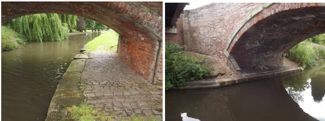
Figure 12 Stone coping at Bridge 106 and replacement stone copings at Bridge 101
