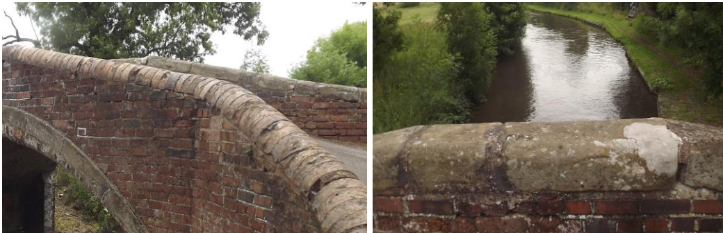
Figure 20 Brick and stone copings to Bridge 105
