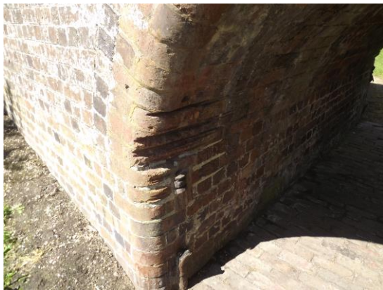
Figure 7 Tow rope wear to bridge 99
