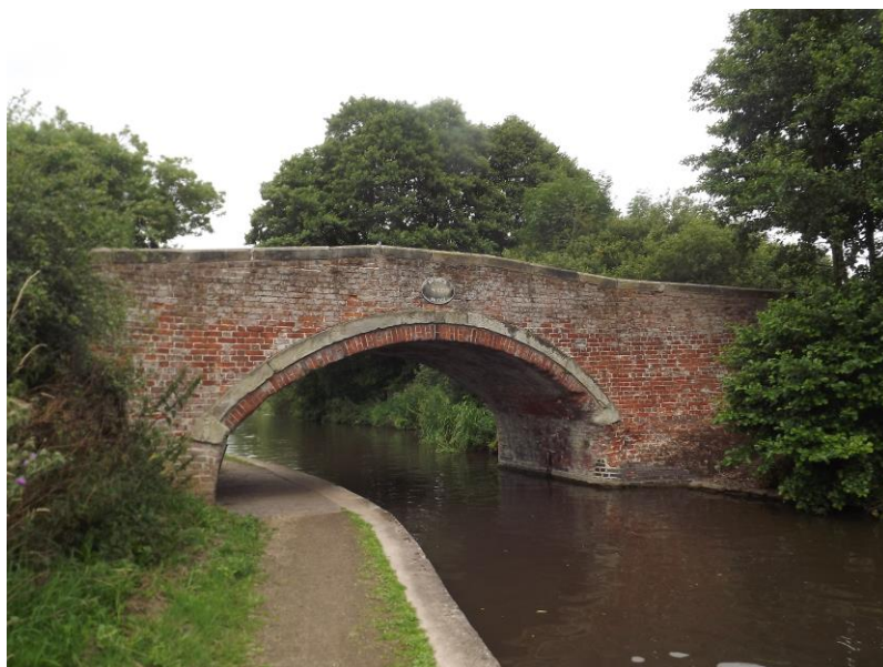
Figure 36 Baswick Bridge, No. 100
