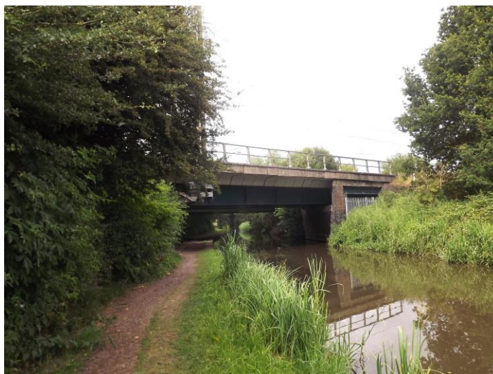
Figure 10 Baswich Railway Bridge 100a
