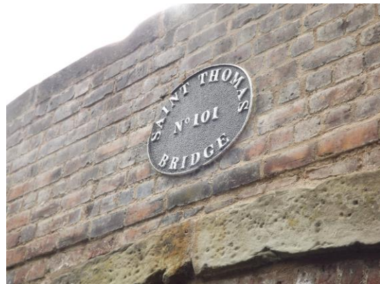
Figure 8 Bridge plate at 101
