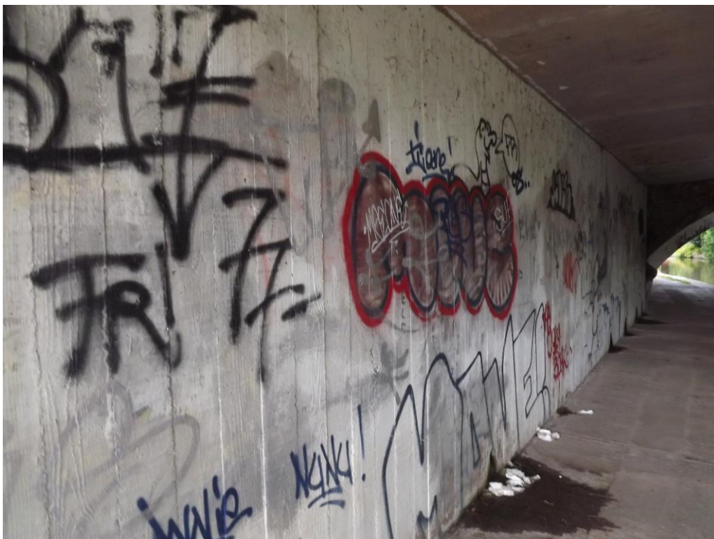
Figure 45 Graffiti at Radford Bridge
