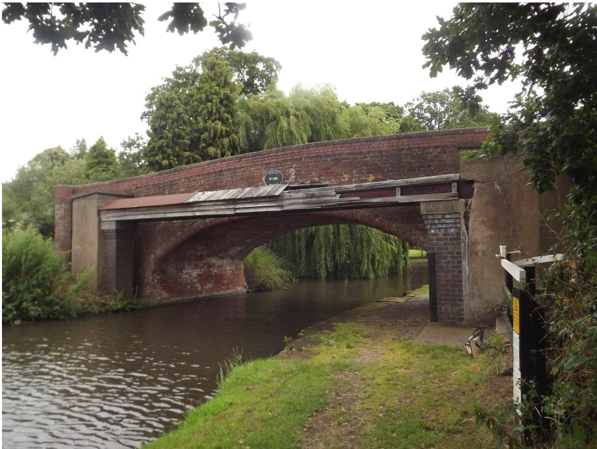
Figure 43 20 th century water pipes and concrete casing at Tixall Bridge
