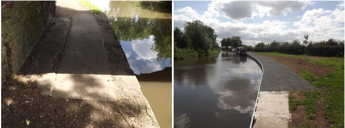
Figure 14 Concrete paving and coping at Bridge 103 and concrete and gravel towpath at Radford
