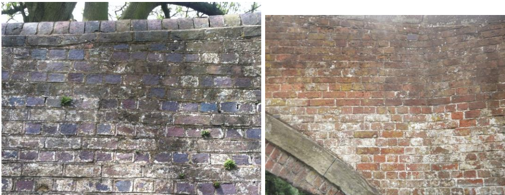
Figure 19 Blue and red brick laid in English Bond to Bridges 104 and 100
