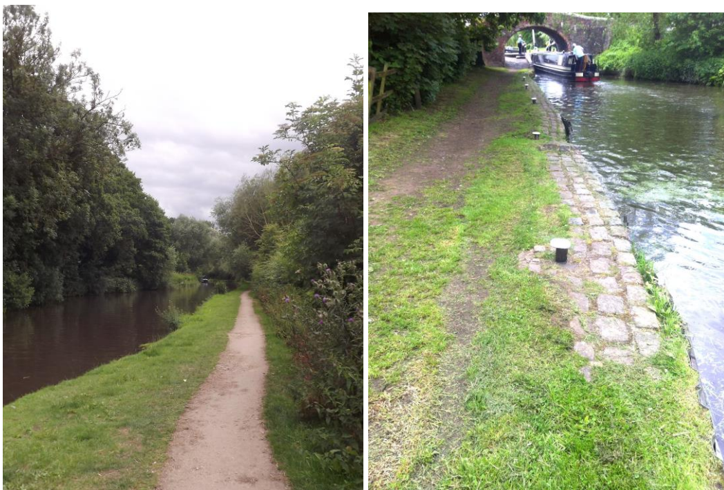
Figure 11 Untreated towpath south of Bridge 100 and brick setts at Bridge 107
