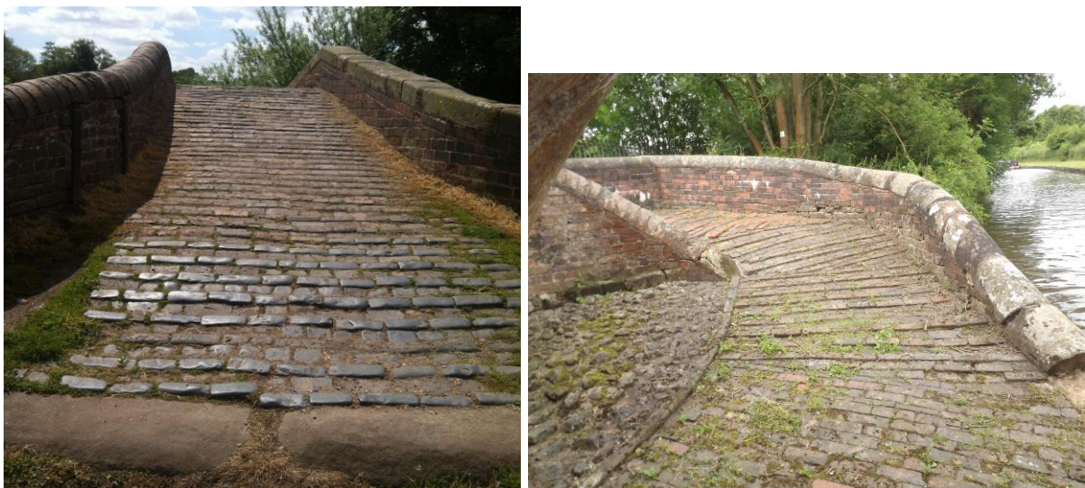
Figure 15 Surviving brick and stone surfacing to Bridges 109 and 105
