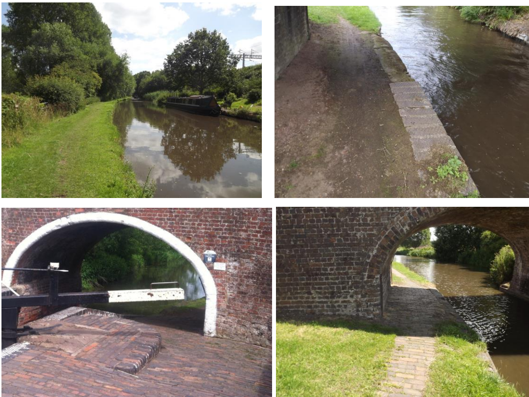
Figure 13 Towpaths are generally untreated although many under bridge sections retain brick and stone setts
