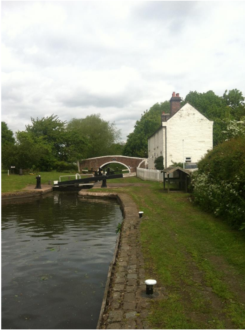
Figure 24 Tixall Lock, Old Hill Bridge and Tixall Lock Cottage
