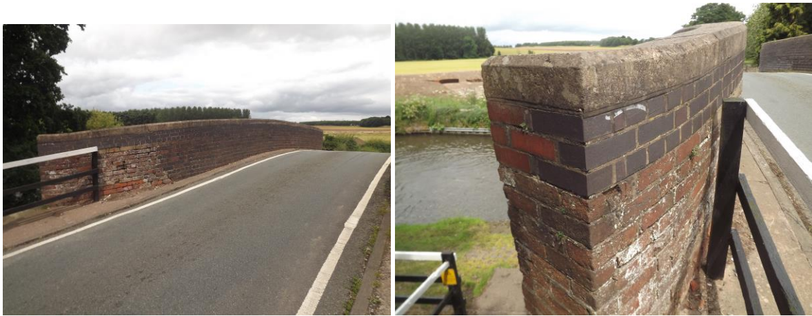
Figure 42 Inappropriate materials at Tixall Bridge
