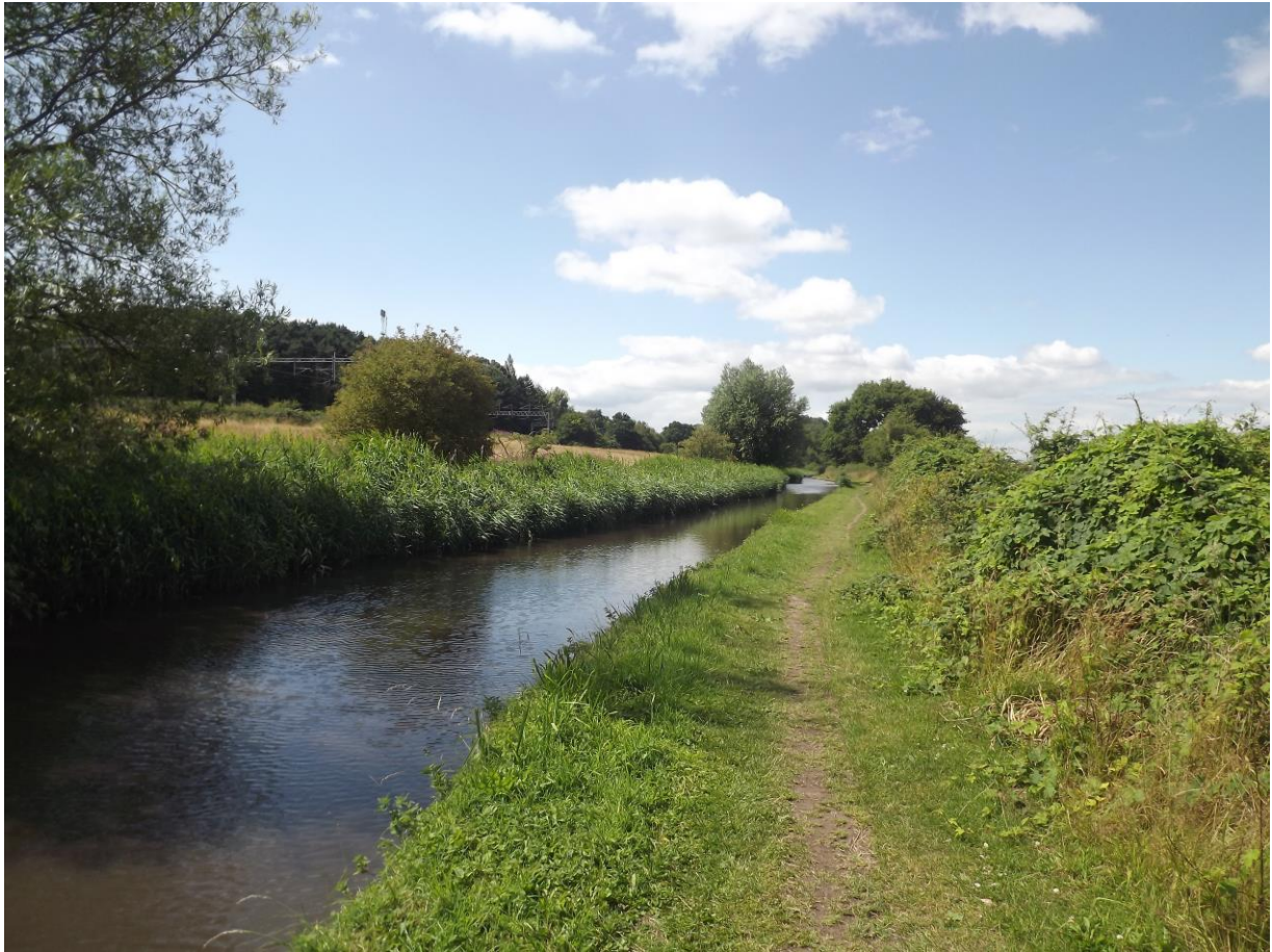
Figure 4 The railway bounds the canal to the south from Milford to Baswich.
