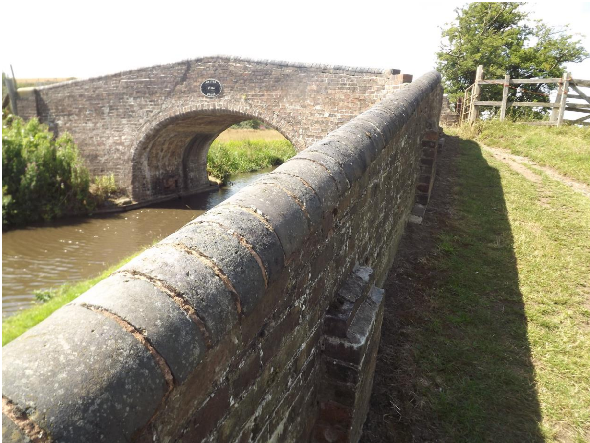
Figure 29 Walton Bridge, No. 104
