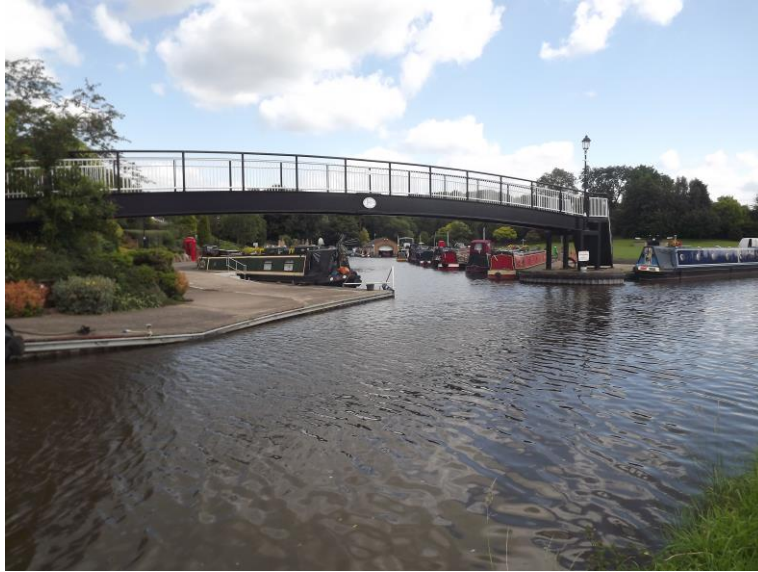
Figure 40 The former Hazlestrine Arm now home to Stafford Boat Club
