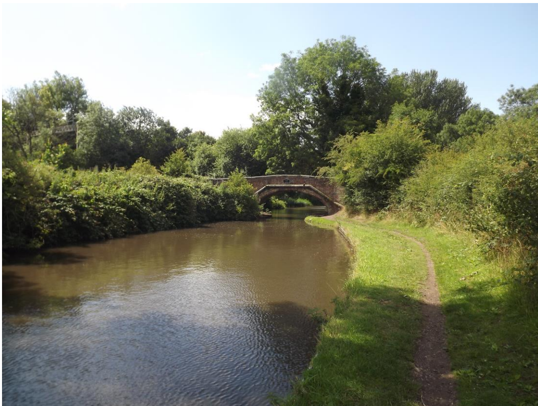
Figure 31 Stoneford Bridge, No. 103
