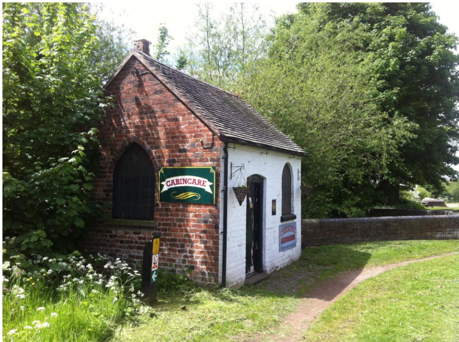
Figure 18 Banksman's lobby at Great Haywood
