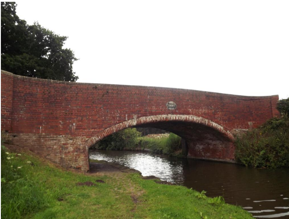
Figure 25 Tixall Bridge, No. 106
