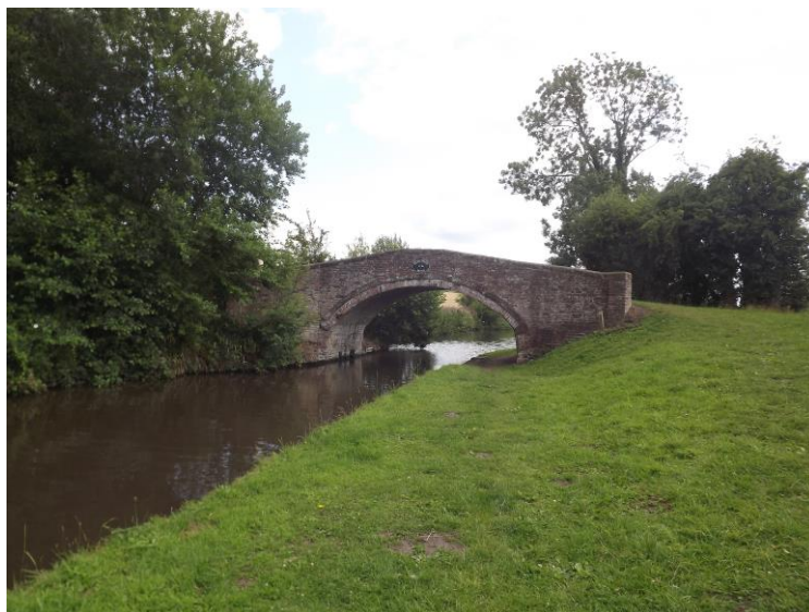
Figure 41 Hazlestrine Bridge, No. 96
