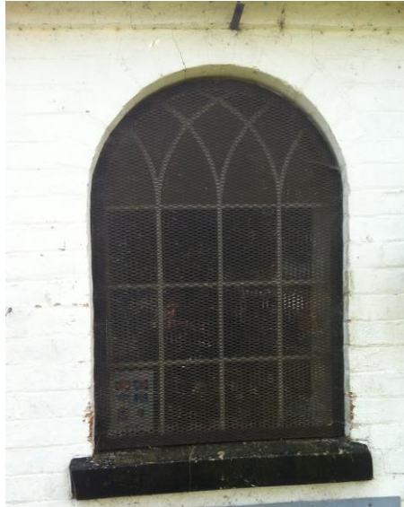
Figure 46 Tracery windows at banksman's lodge obscured by security grilles
