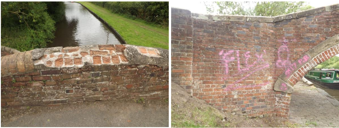
Figure 44 Vandalism and graffiti at Milford Bridge
