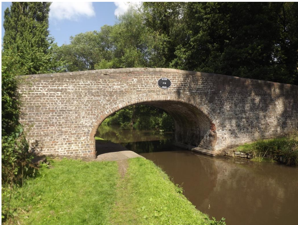
Figure 37 Meadow Bridge, No. 99
