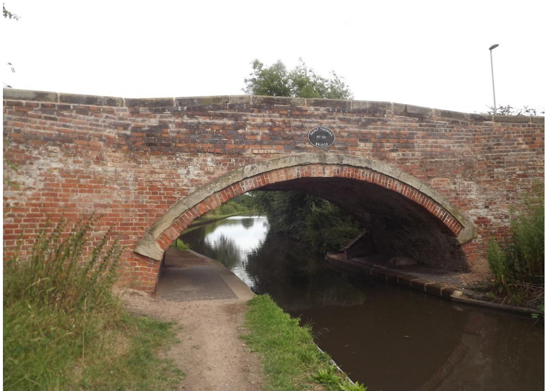
Figure 33 The grade II listed Saint Thomas Bridge (No.101)
