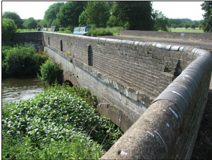
Figure 9 Aqueduct over the River Trent
